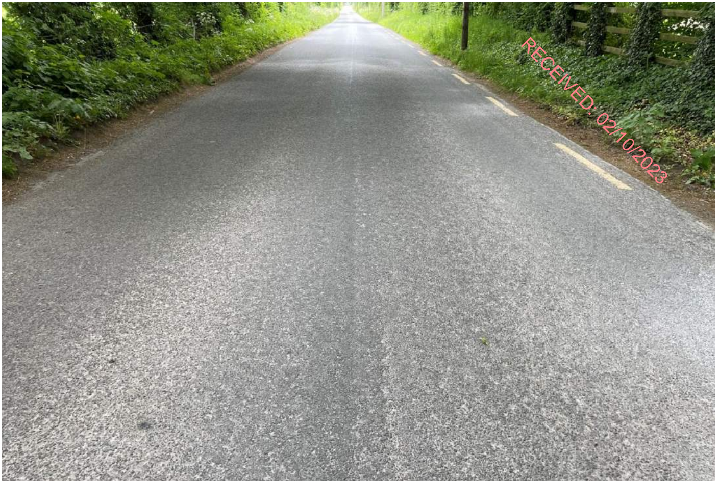
Picture B13: Section C – Chainage 2800
