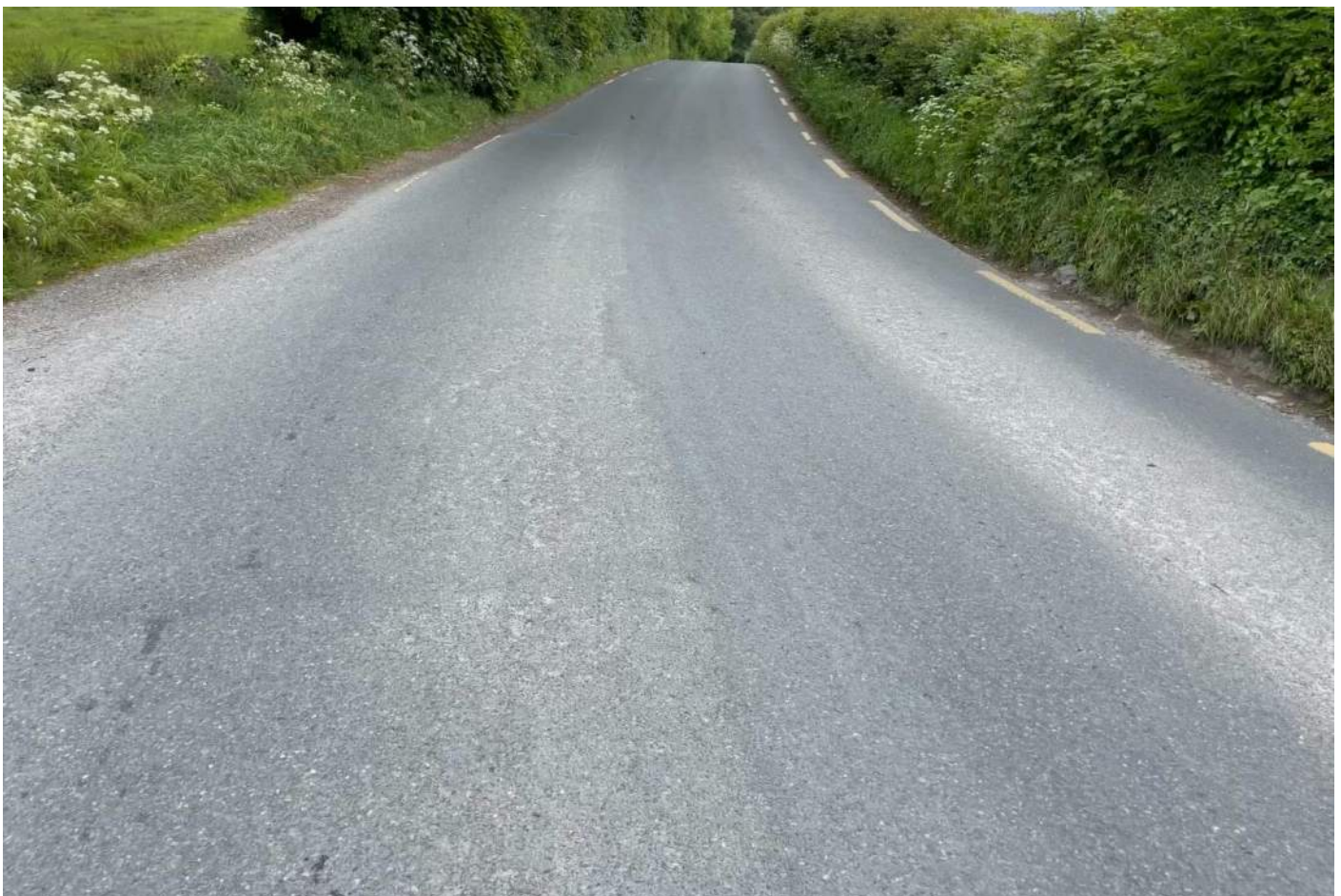
Picture B8: Section B – Chainage 1200
