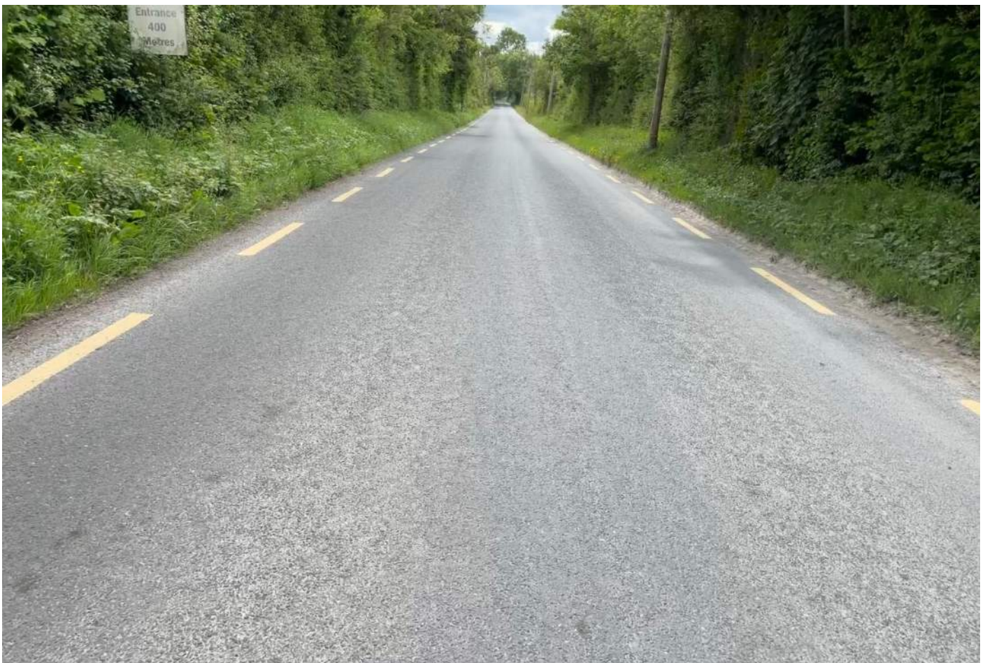
Picture B14: Section C – Chainage 3120
