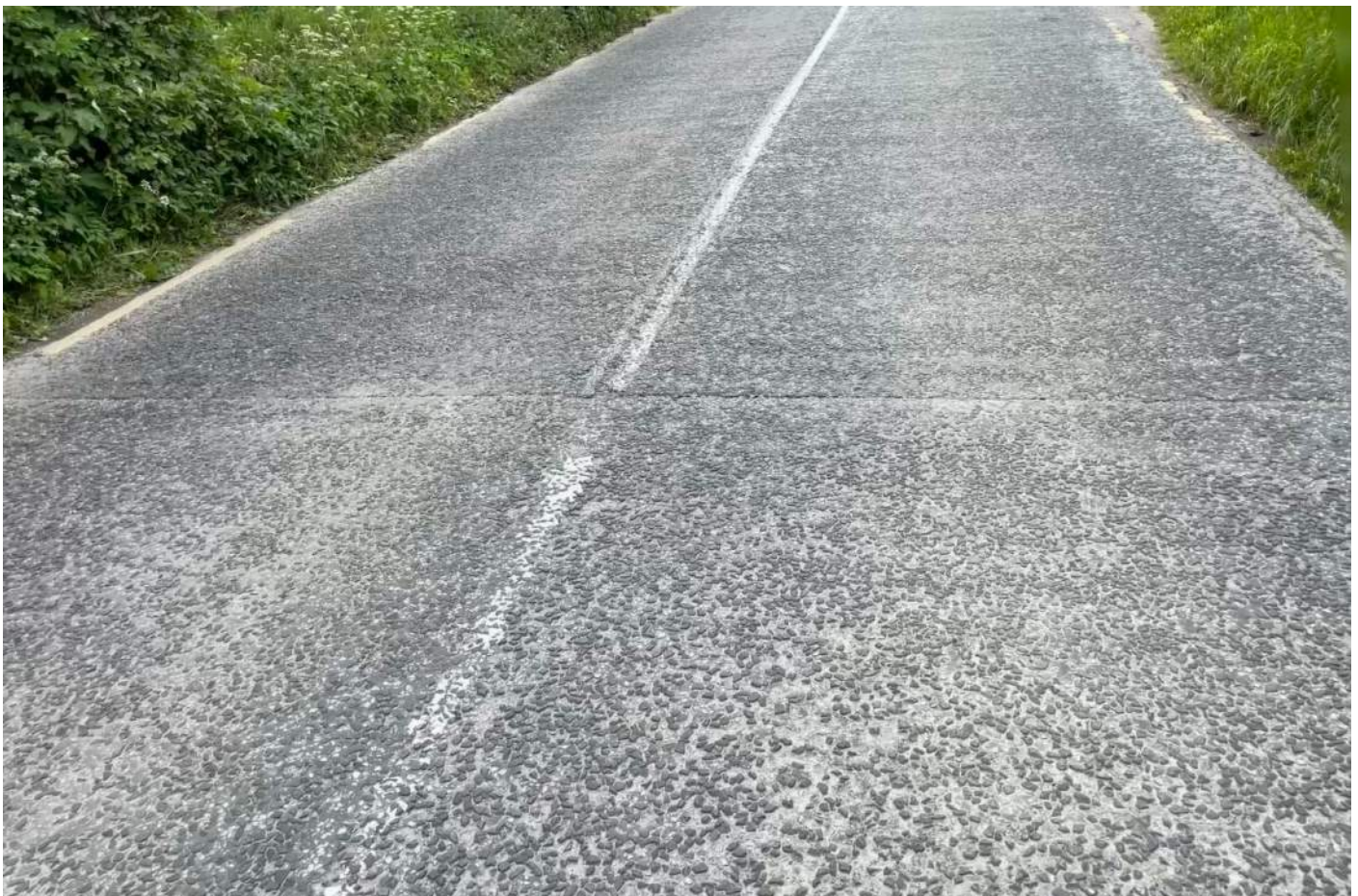
Picture B4: Section A – Chainage 215 – Transverse Joint in HRA
