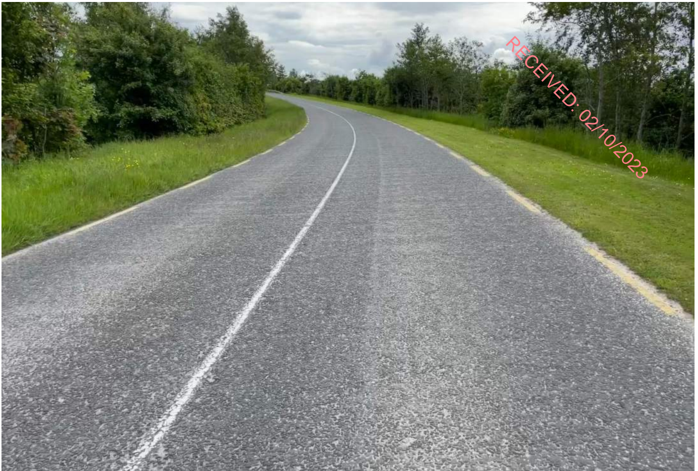
Picture B5: Section A – HRA Surface approaching Motorway Bridge
