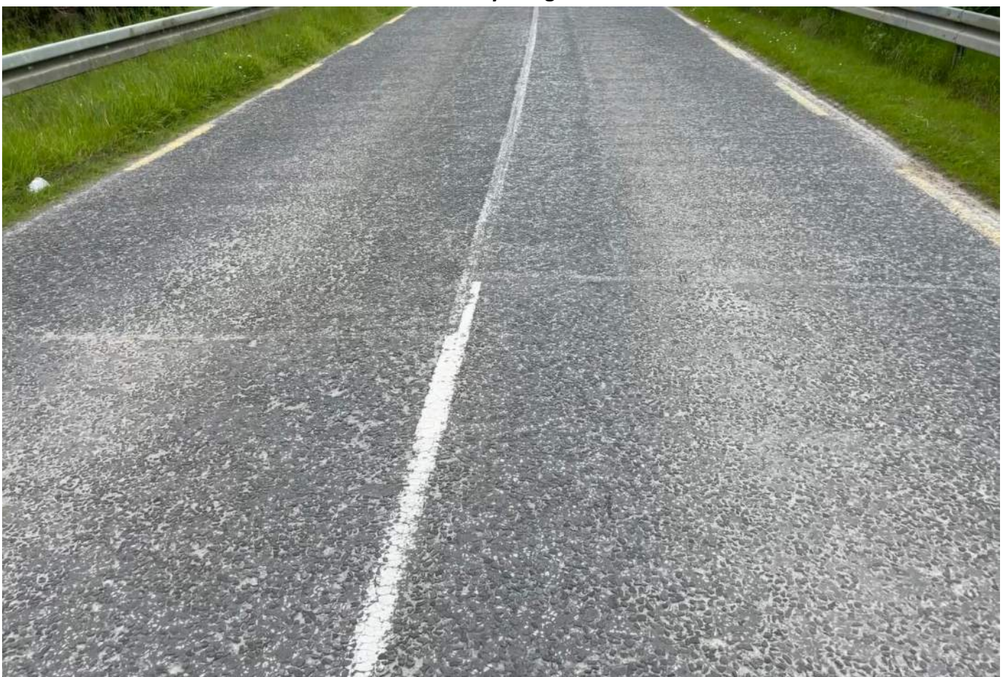
Picture B6: Section A – HRA Joint south of Motorway Bridge
