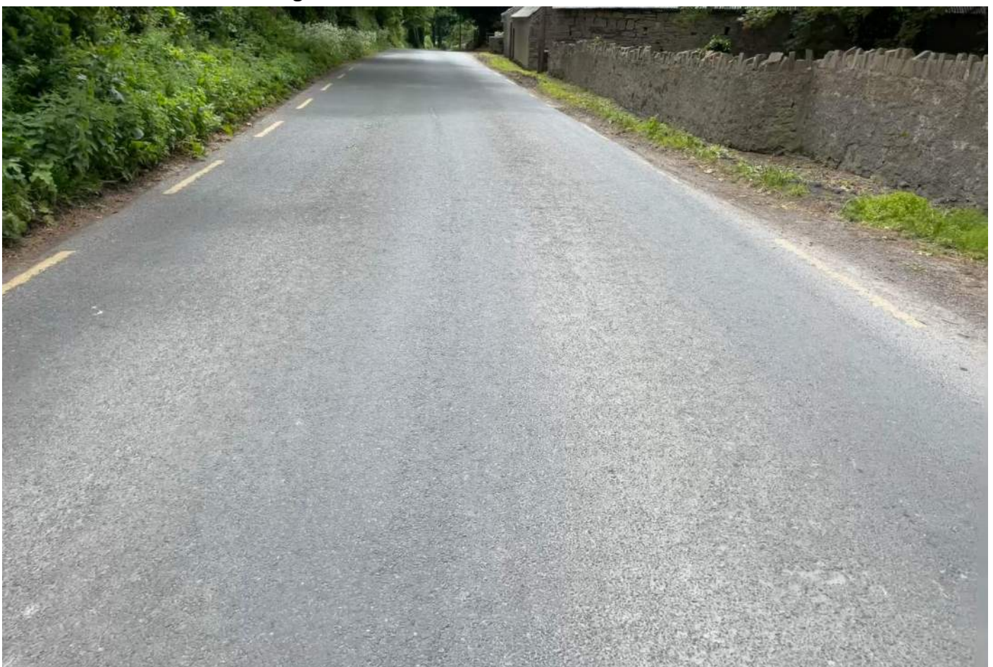
Picture B12: Section B – Chainage 2600
